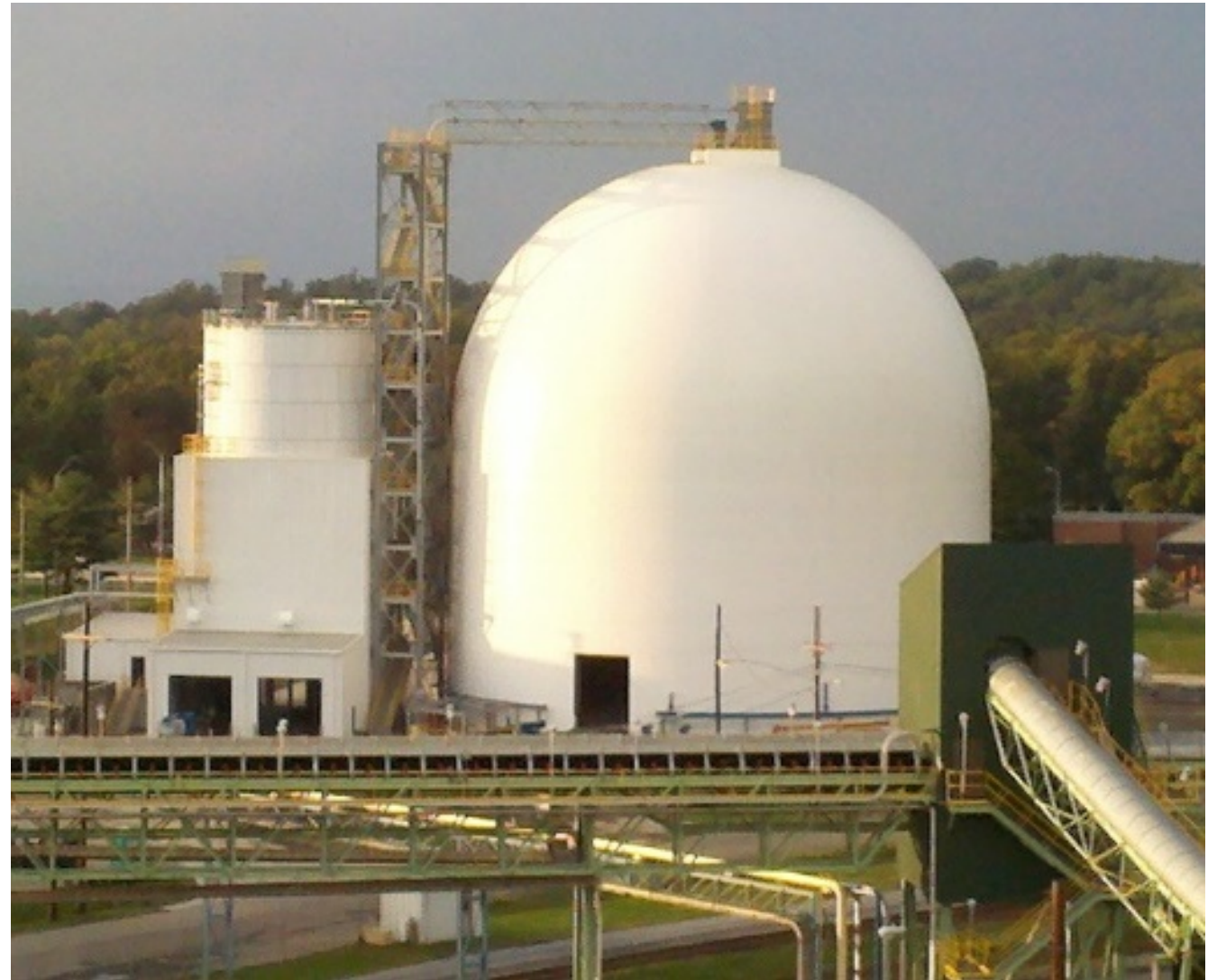
30,000 ton Dome & Dual Enclosed Load Out
